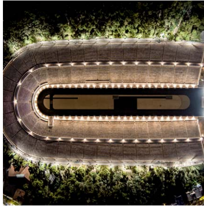
Panathenaic Stadium (Athens / Greece)
