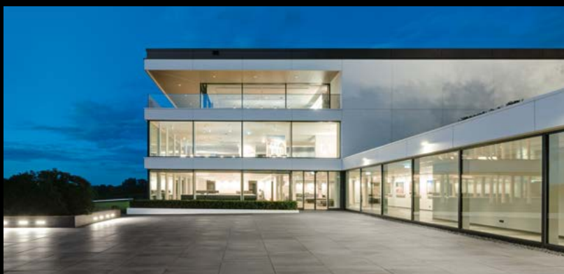
The BEGA Competence Center in Menden offers a comprehensive insight into our portfolio of high-quality luminaires and design elements for virtually any application.
